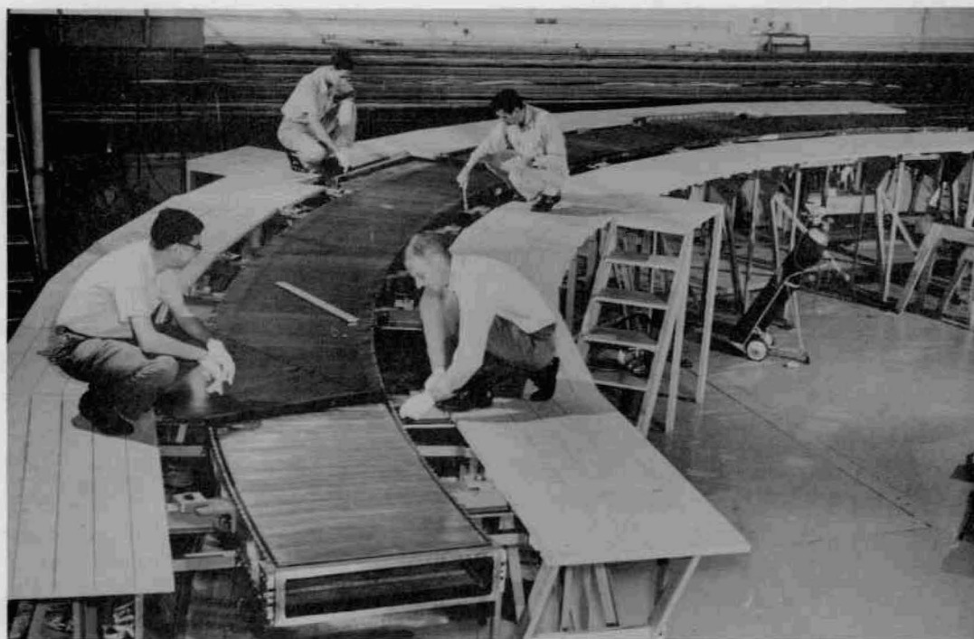
Figure 6. The first quadrant, now almost completely assembled, of the vacuum chamber of the Cosmotron. Stainless steel, 1-in thick, side walls support a grid of stainless steel bars, 2-in wide. Over this grid, top and bottom, is stretched an airtight sheet of Myvaseal rubber.
