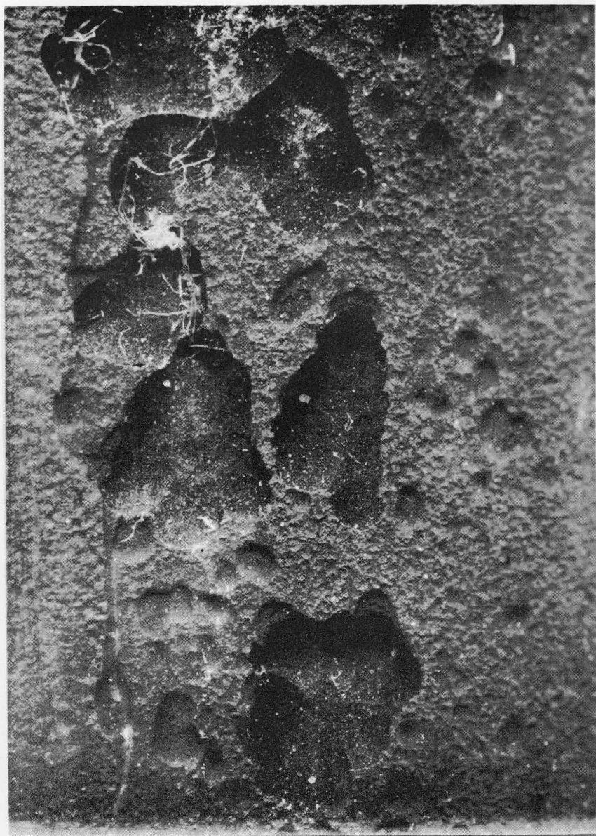
Fig. 55 Feed Stream Pipe Pitted Area 11 ft from Outlet (Hot) End (15X)
