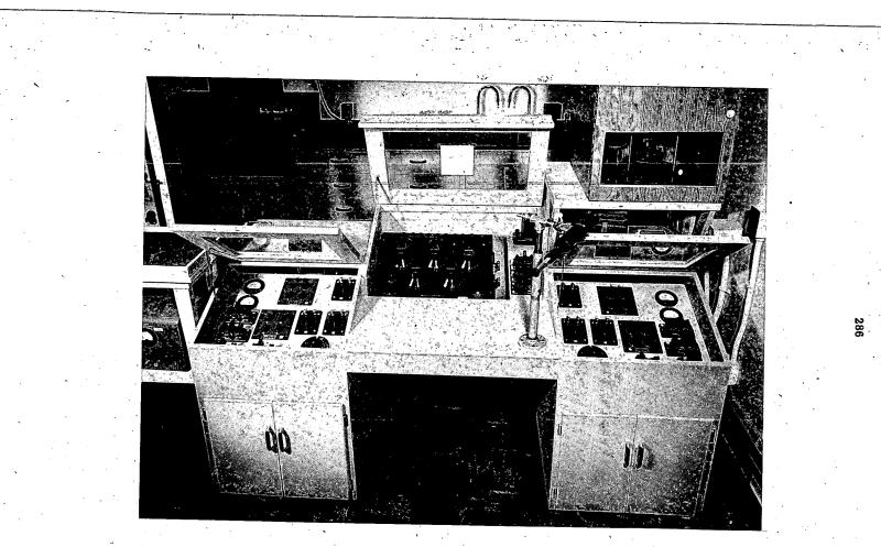
Fig. 10.5 — Typical calorimeter console.
