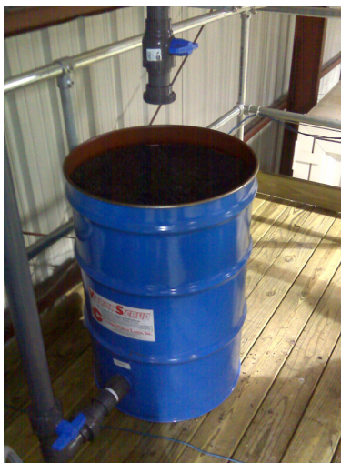
Figure 8: 200 lbs charcoal column from Cameron Carbon Inc.
