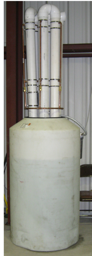
Figure 7: Water mist air filter installed at KURF
