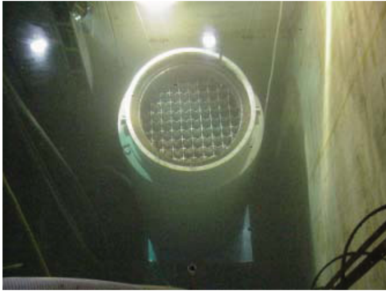
Figure G2-2. Holtec International cask in fuel storage pool). Figure taken from Holtec International Web site.
