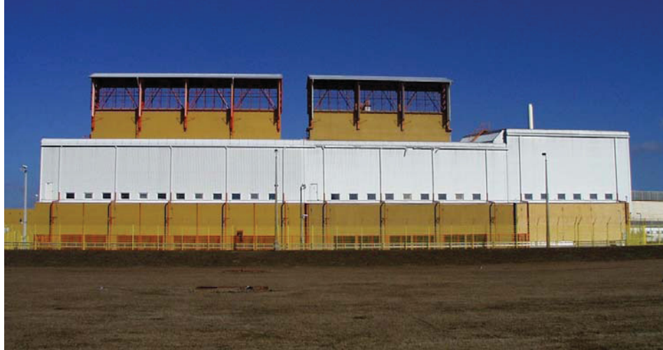
Figure E4-6. Paks MVDS in 2000 showing natural convection cooling exhaust outlets (Ordogh et al. 2004).
