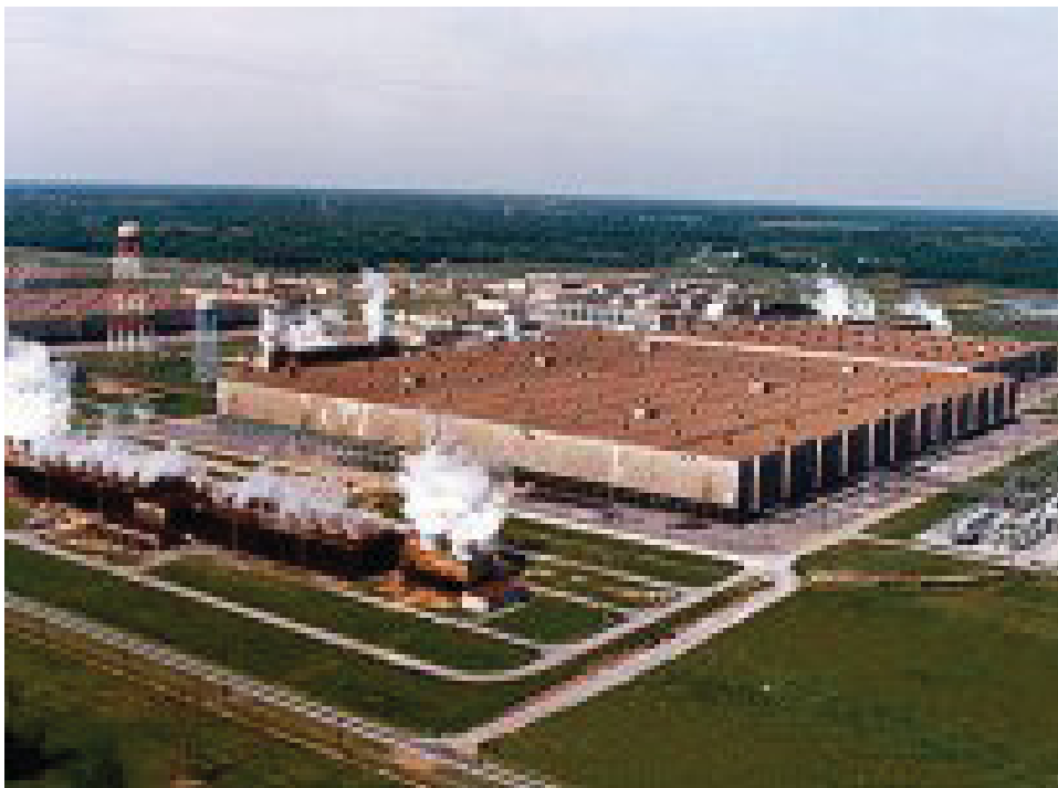
Figure C1-8. United States Enrichment Corporation Gaseous Diffusion Production Building.
