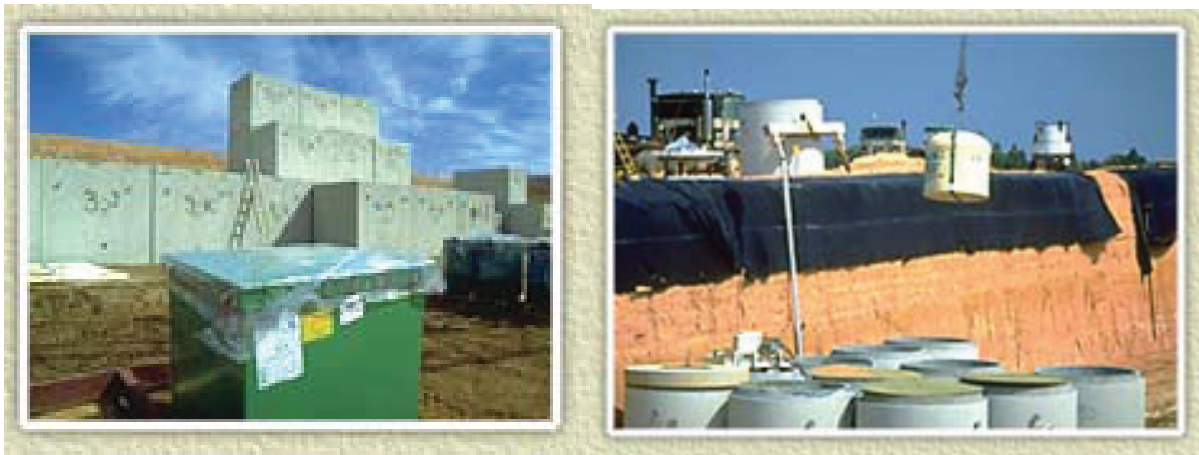
Figure G3-5. Waste placement in landfill at Chem-Nuclear Systems Barnwell site (Chem-Nuclear Systems, LLC 1997).
