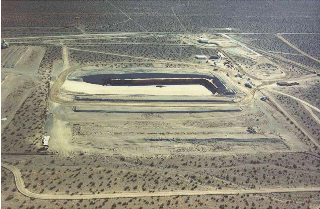
Figure J-3. Nevada Test Site low-level waste disposal facility aerial view (State of Nevada 2009).
