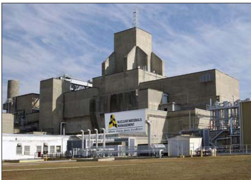
K-Area Materials Storage Facility at SRS
