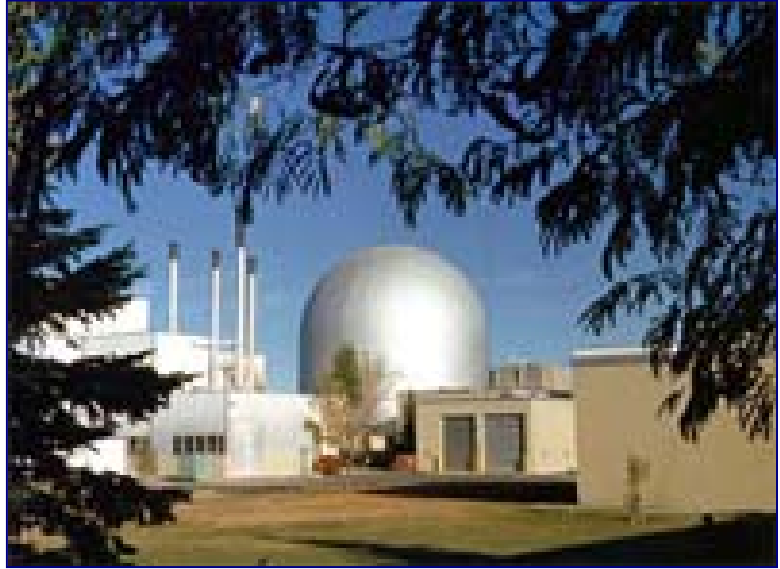
Experimental Breeder Reactor-II containment dome
