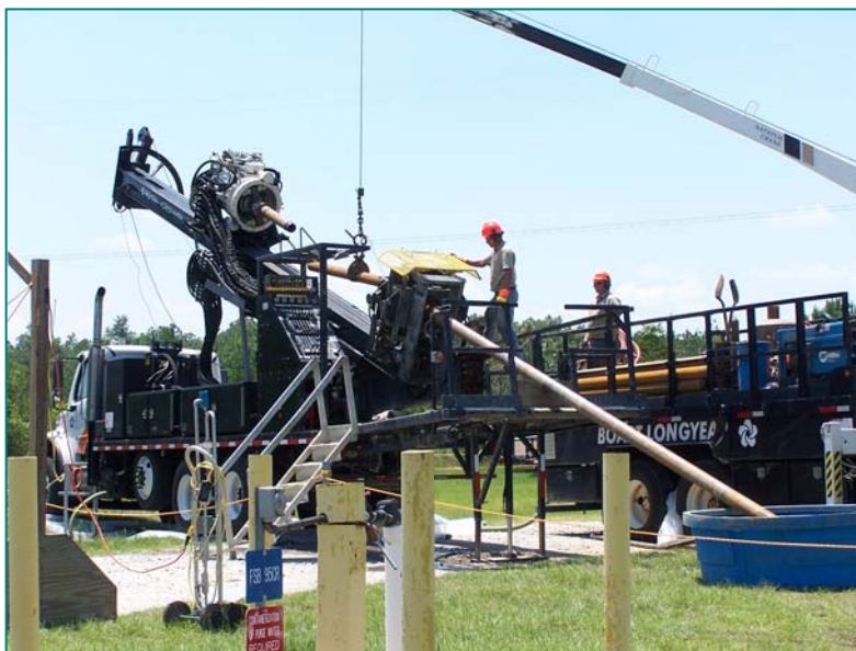
Diagonal drilling beneath F-Area seepage basin to support sampling
