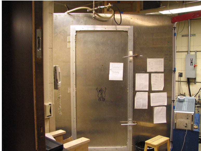
Figure 2.7: Image of current generation magnetic shield. The shield weighs approximately 1 ton, and is constructed of 6mm thick aluminum plates bolted with brass bolts to an aluminum frame.
