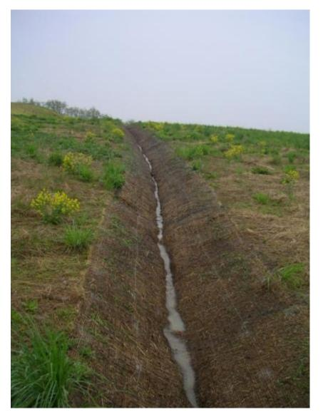
Figure 8 – Stormwater Diversion Ditch to Collect Offsite Water
