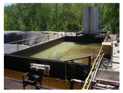
Figure 25 – Settling Tank – Pennsylvania Brine
