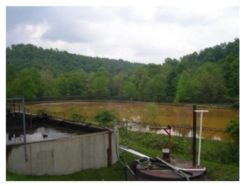
Figure 31 – Aeration Tank – with and without Anti-Foaming Chemical – Tunnelton Liquids
