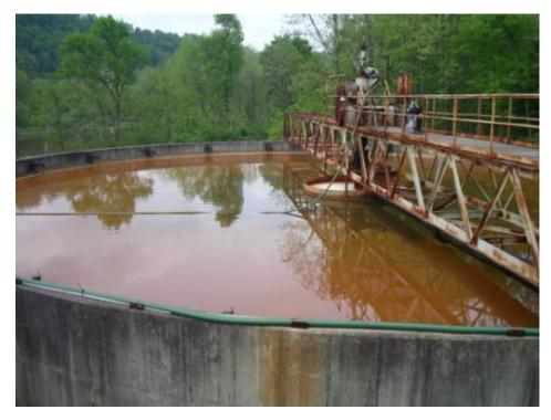
Figure 32 – Clarifier – Tunnelton Liquids
