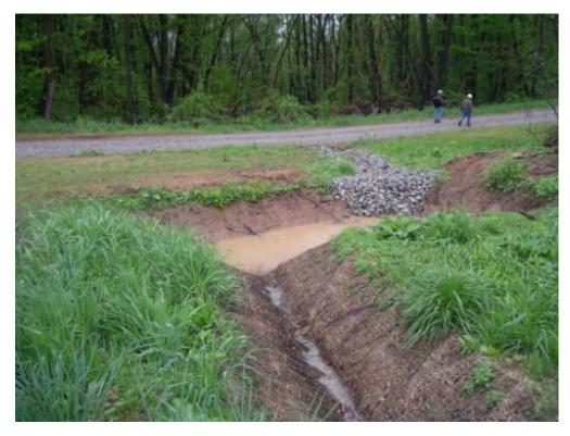
Figure 9 – Lower End of Stormwater Diversion Ditch
