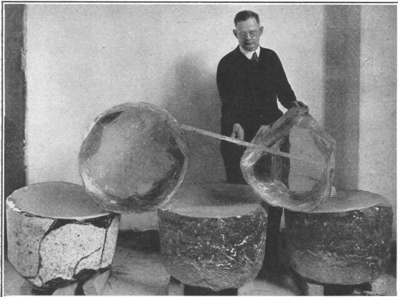
FIG. 21.— High-grade optical glass produced at bureau
