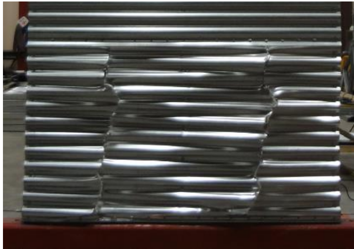
Figure 35. Failure mode of wall configuration Type 9
