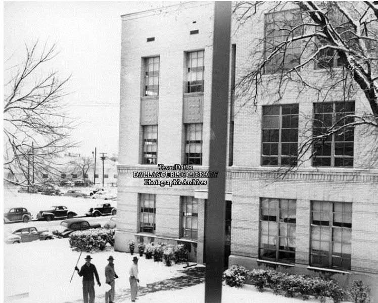
Figure 4.3. Crozier Technical High School, 1950. Photo courtesy of the Dallas Public Library, Texas/Dallas History and Archives Division.
