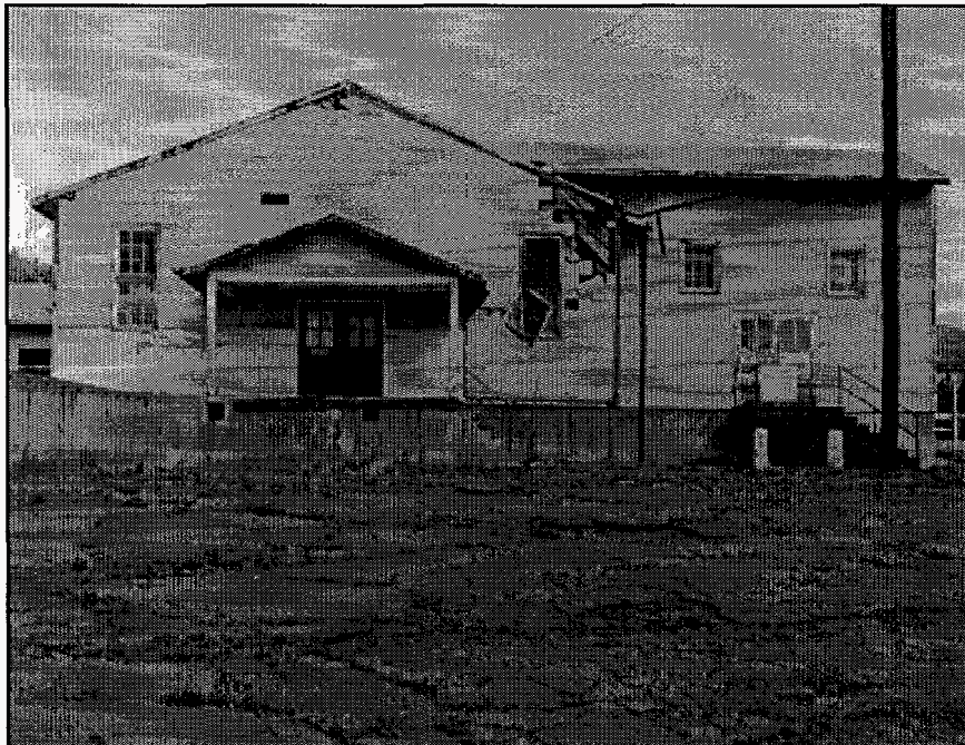
Figure 4a. Building TA-16-27, east side of casting facility
