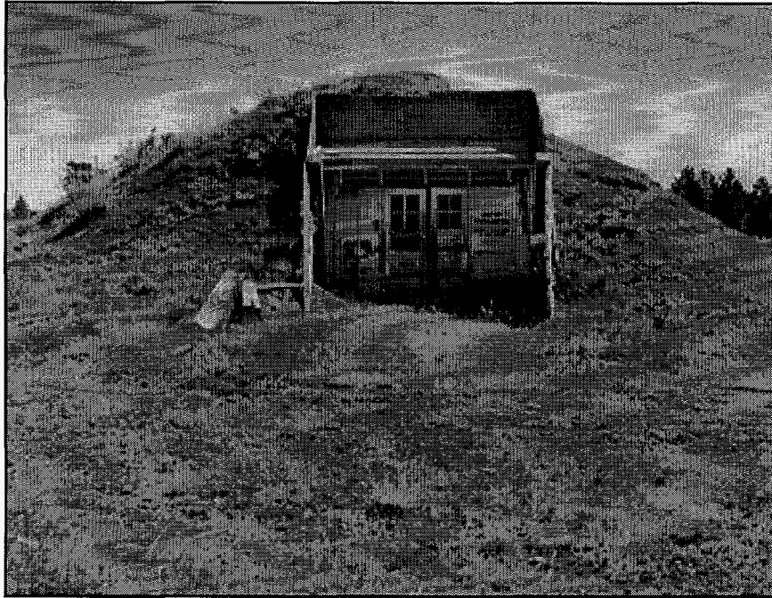
Figure 3. Building TA-16-77, concrete bunker with earthen barricade
