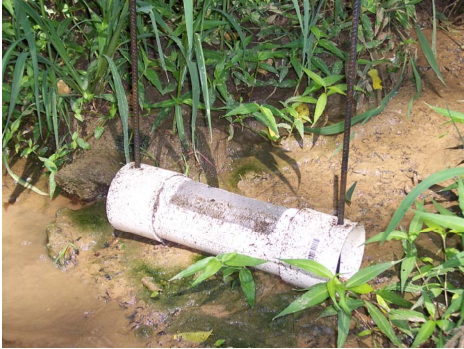
Fig. 7. Photograph showing cage construction.
