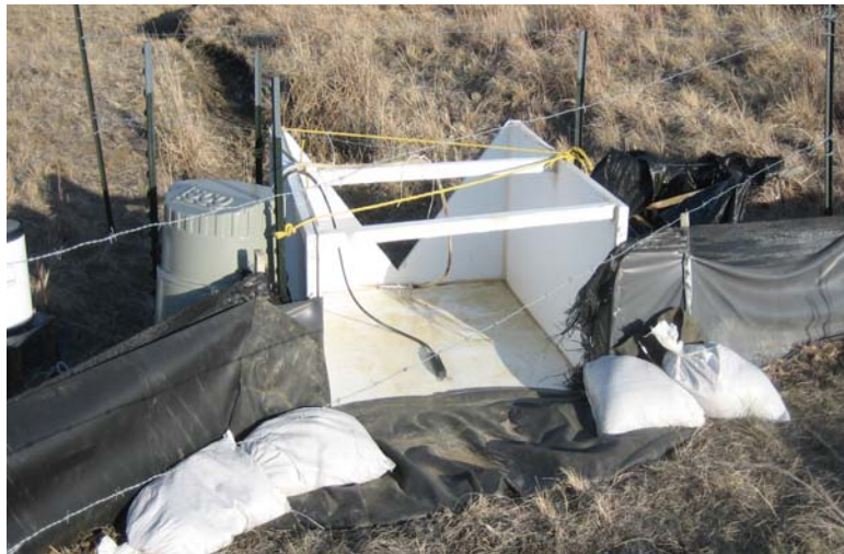
Figure 7. Weir design. A 90° v-notch weir with barrier fencing, a gray ISCO™ sampler, ground plastic, and sand bags to stop undercutting. Equipment is enclosed in barbed wire fencing to prevent cattle disturbances.
