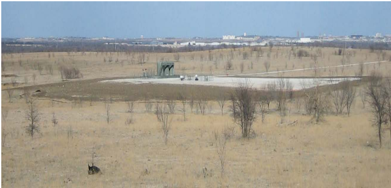
Figure 6. Typical gas well site. A filter berm was used to prevent erosion and can be seen as the thin black line running through the grass along the edge of the disturbed area.
