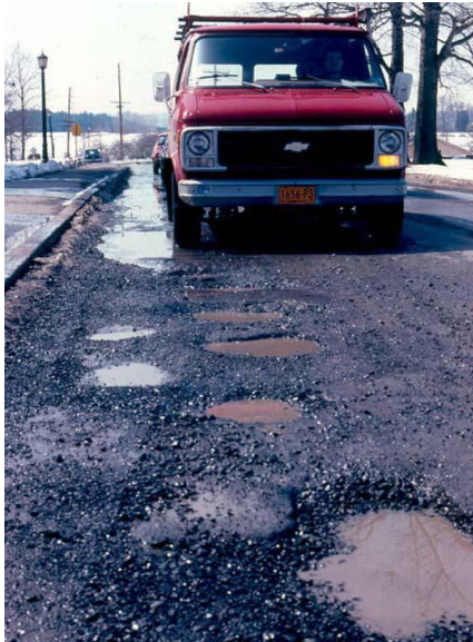
Figure 10: Potholes Courtesy: Kearney, E.J. et al. 2004
