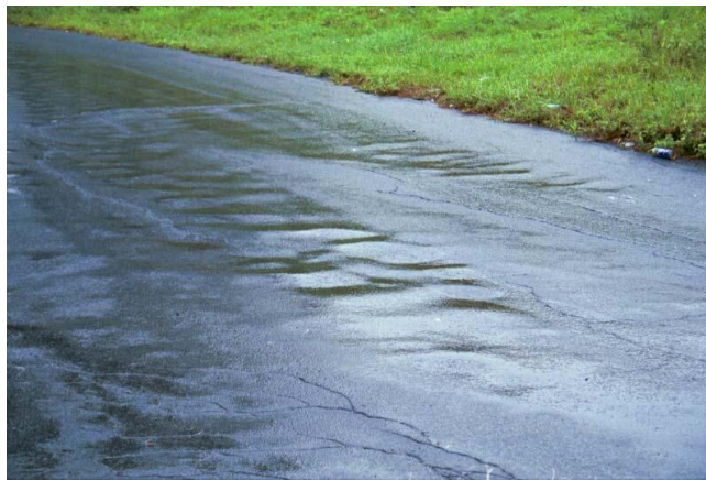
Figure 9: Shoving Courtesy: Kearney et al. 2004
