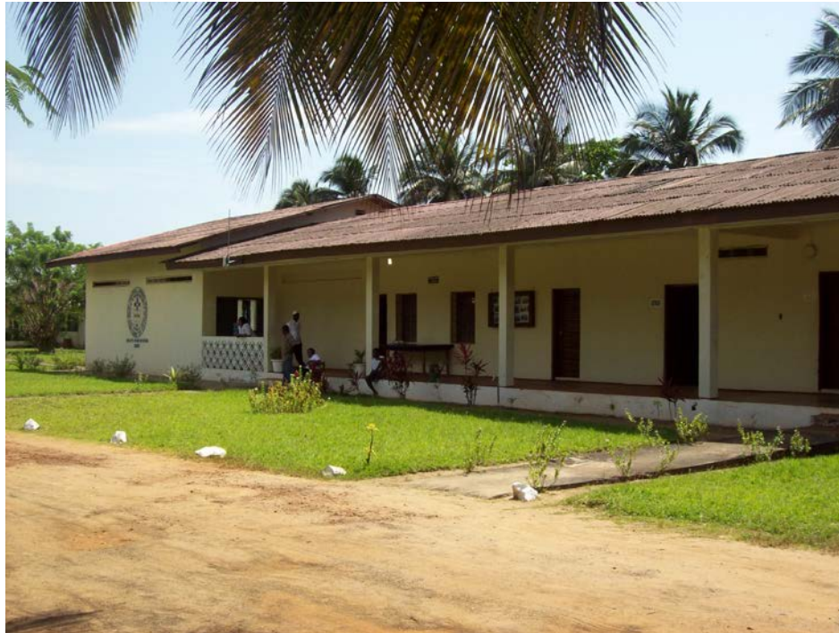
Figure 14. Partial view of the Administrative Building.
